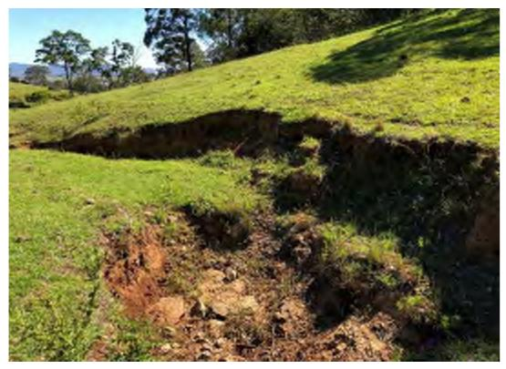
Photograph 39: View of heavy erosion of spill way on Dam West
