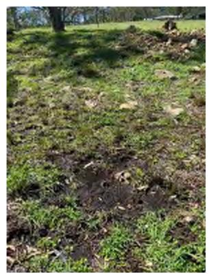
Photograph 5: View looking south east at the northern wall of Dam South showing dam seepage
